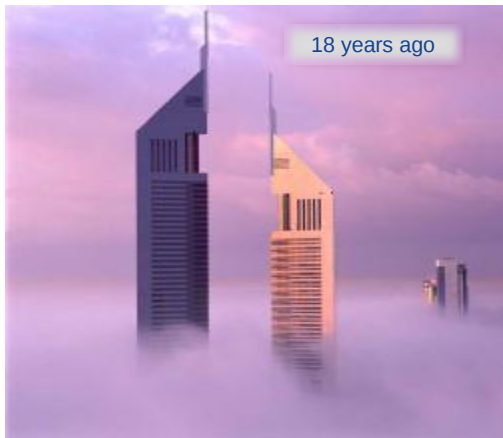
Emirates Tower Hotel Dubai, UAE Completed 1999 309 m, 22 Floors Thermalbond V2200 Series
